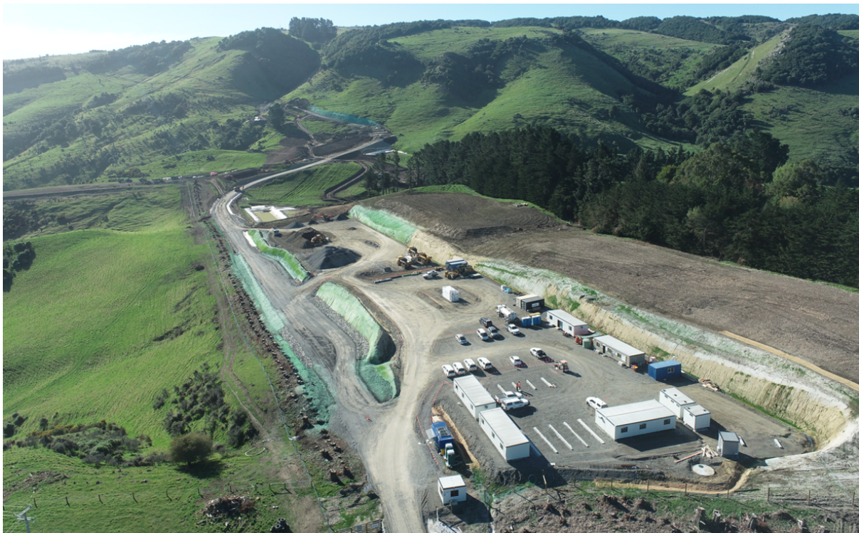
Figure 5 Site Construction Camp
