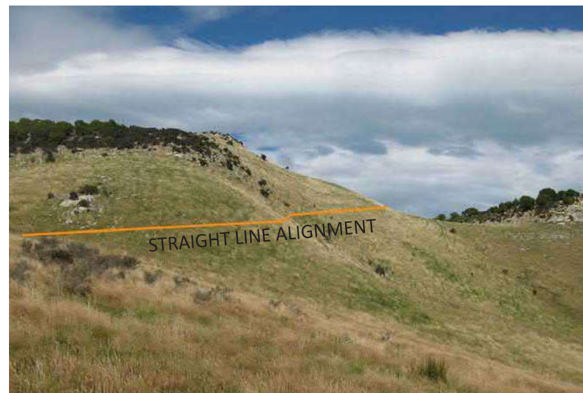
Fig. 5 Before: Straight line alignment of road.
