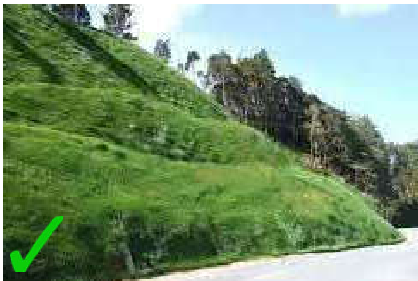
Fig. 39 Avoid benching in even steps.
