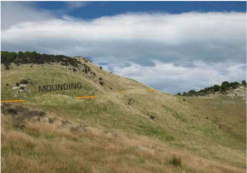
Fig. 7 After: Add fill material to create mounds or vegetation to reduce impact of road.
