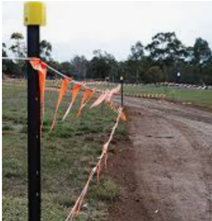
Figure 1 Exclusion Zone Fencing
