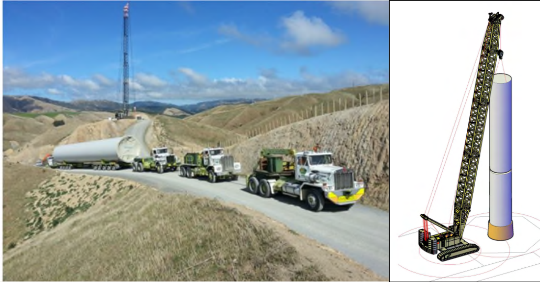
Figure 19 Example of Tower Section Delivery from a Historic Project
