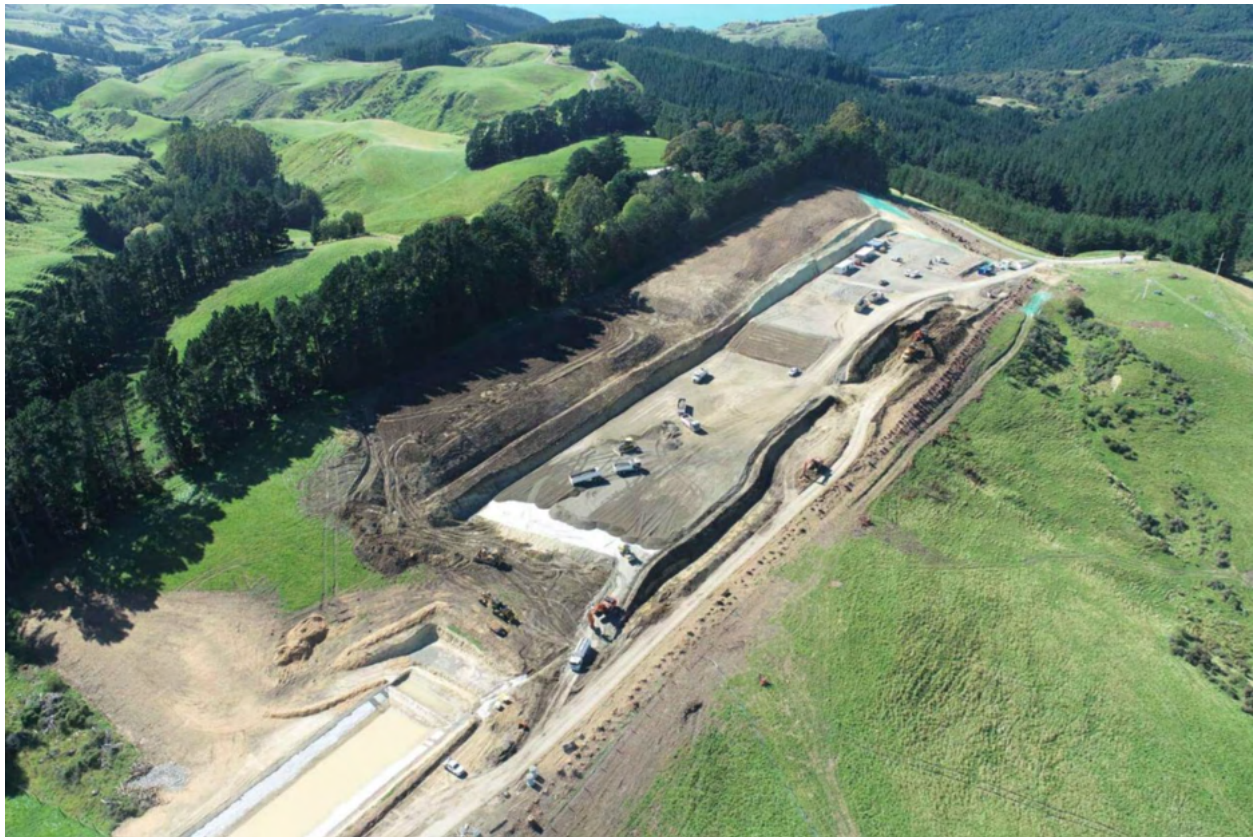
Figure 10- Site Office and aggregate laydown area (March 2026)
