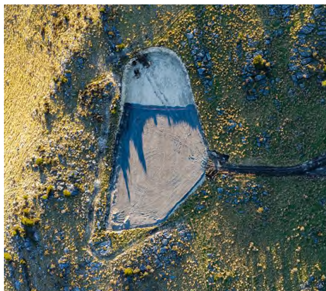
Turbine pad area of Wind Turbine 3
